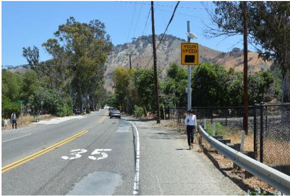
Figure 4: Highway 33 does not have dedicated pedestrian space along the roadway.
