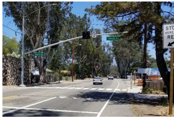
Figure 1: Pedestrian crossing infrastructure at Ranch Road.
