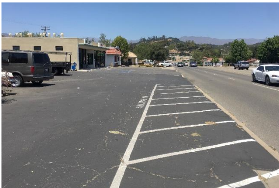
Figure 8: Options for pedestrians in study area extremely limited, such that they are forced to use the asphalt of a parking lot as a walkway.
